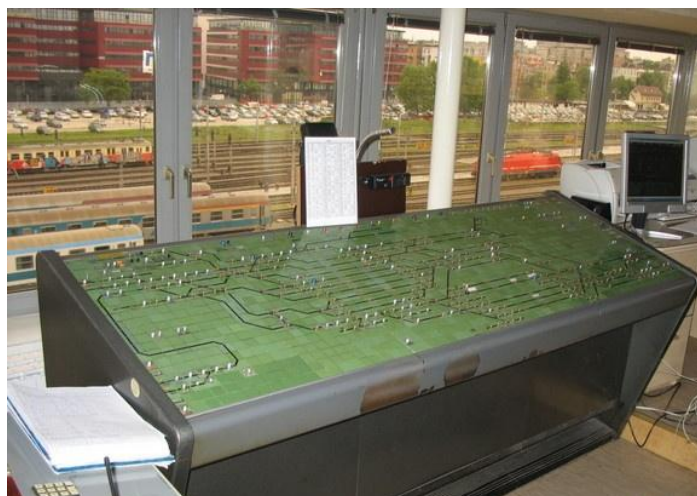
Slika 18: Postavljalna miza (Vir: http://img516.imageshack.us/img516/3750/picture006fs3.jpg )
