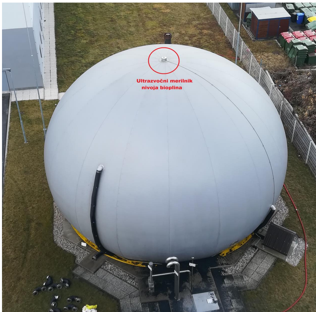
Slika 10: Obstoječi plinohram 1000 m 3 v CČN Kranj (Vir: Lastni, december 2018)
