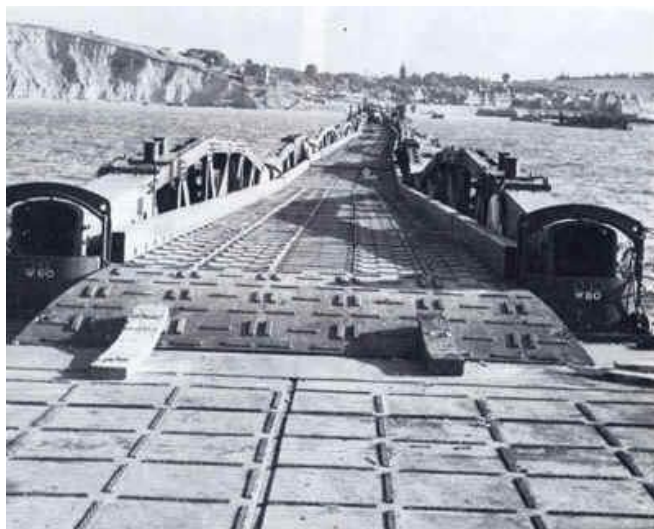
Slika 7: Pontonski most (Vir: The Mulberry Harbour, 2015)
